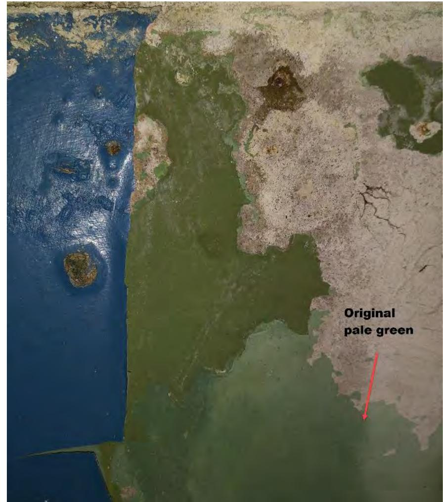
Plate 41: Original paintwork colour identified in the eastern rear stairs.
