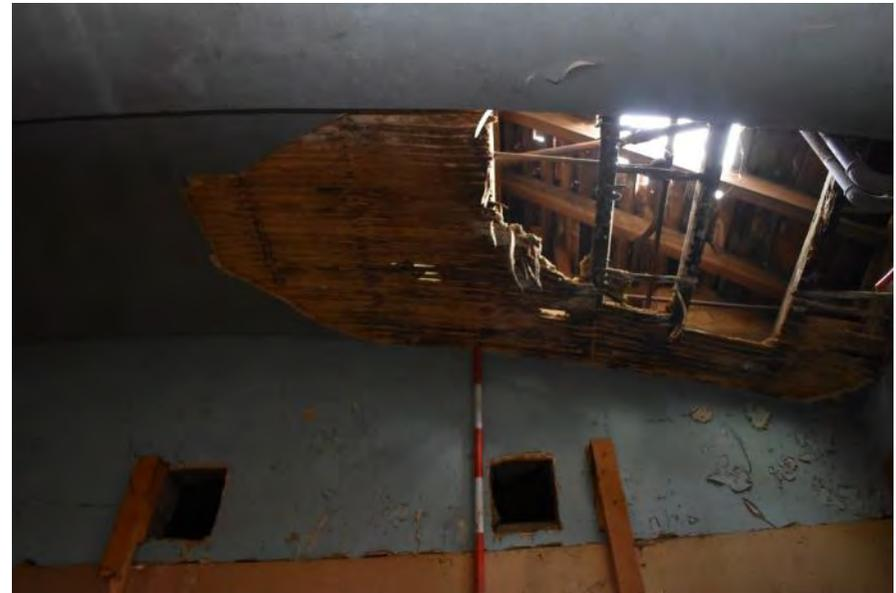
Plate 55: Roof open to the elements in first floor room (facing W)
