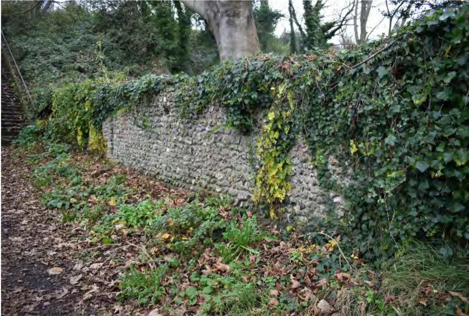
*Plate 30: Flint wall on the southern boundary of the churchyard. Example of likely construction within PDA as well. (facing NW)*
