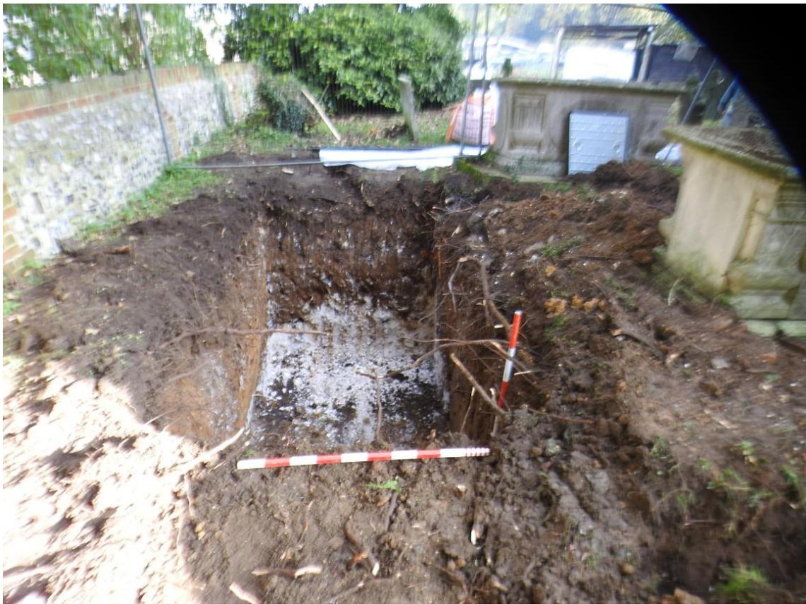
Plate 9. Excavation for new septic tank
