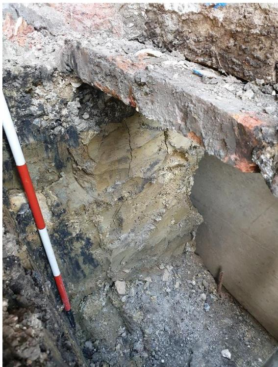
Photo 10. Slag foundation base (red arrow)
