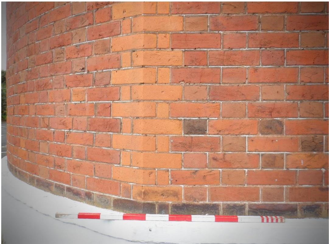
Plate 10. Brick details of corner built with splayed bricks set with Flemish Bond courses
