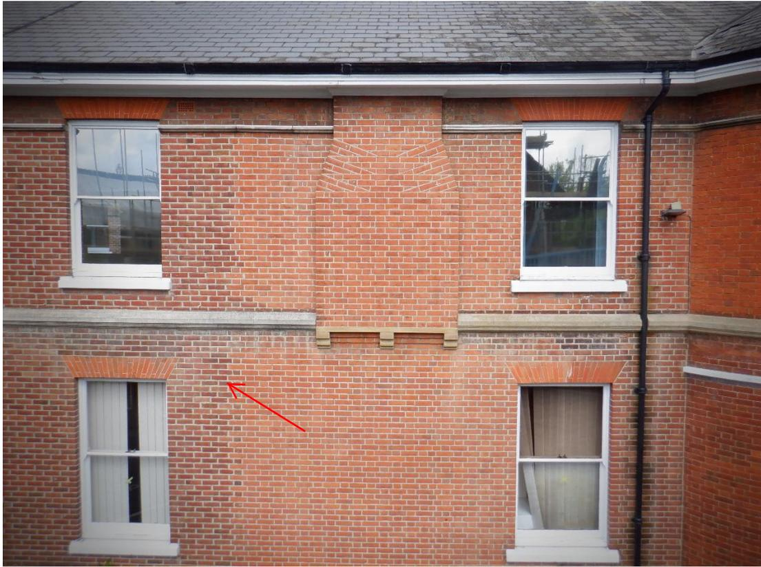
Plate 20. Detail of later south-east build to the left and red arrow marks the join
