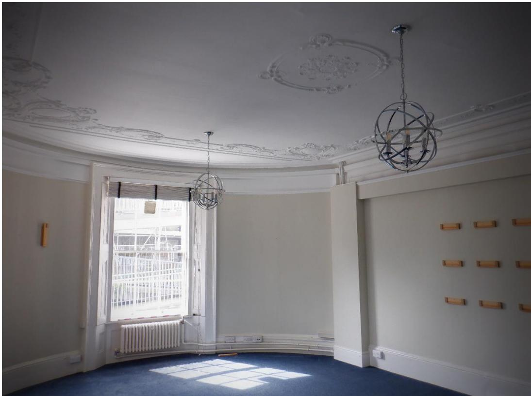
Plate 42. Plaster decoration with ceiling rose, coving, cornice and panel moulding
