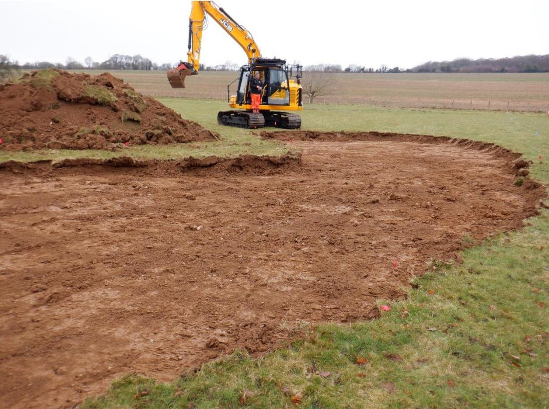
Plate 3. Topsoil strip (looking North)
