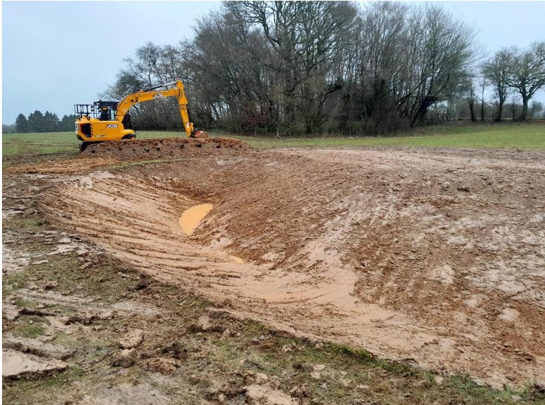
Plate 5. Completed soil strip and reduction (looking North)
