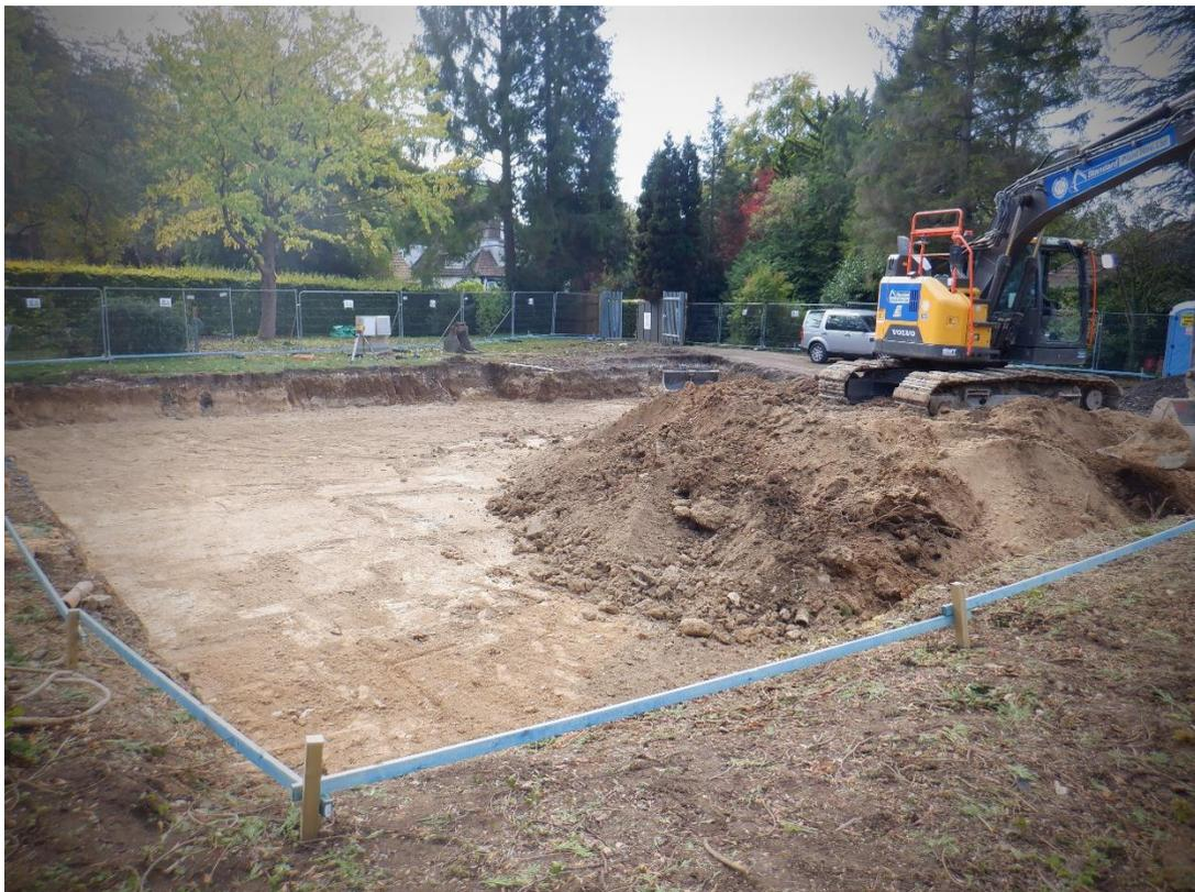
Plate 6. Ground reduction (looking NW)
