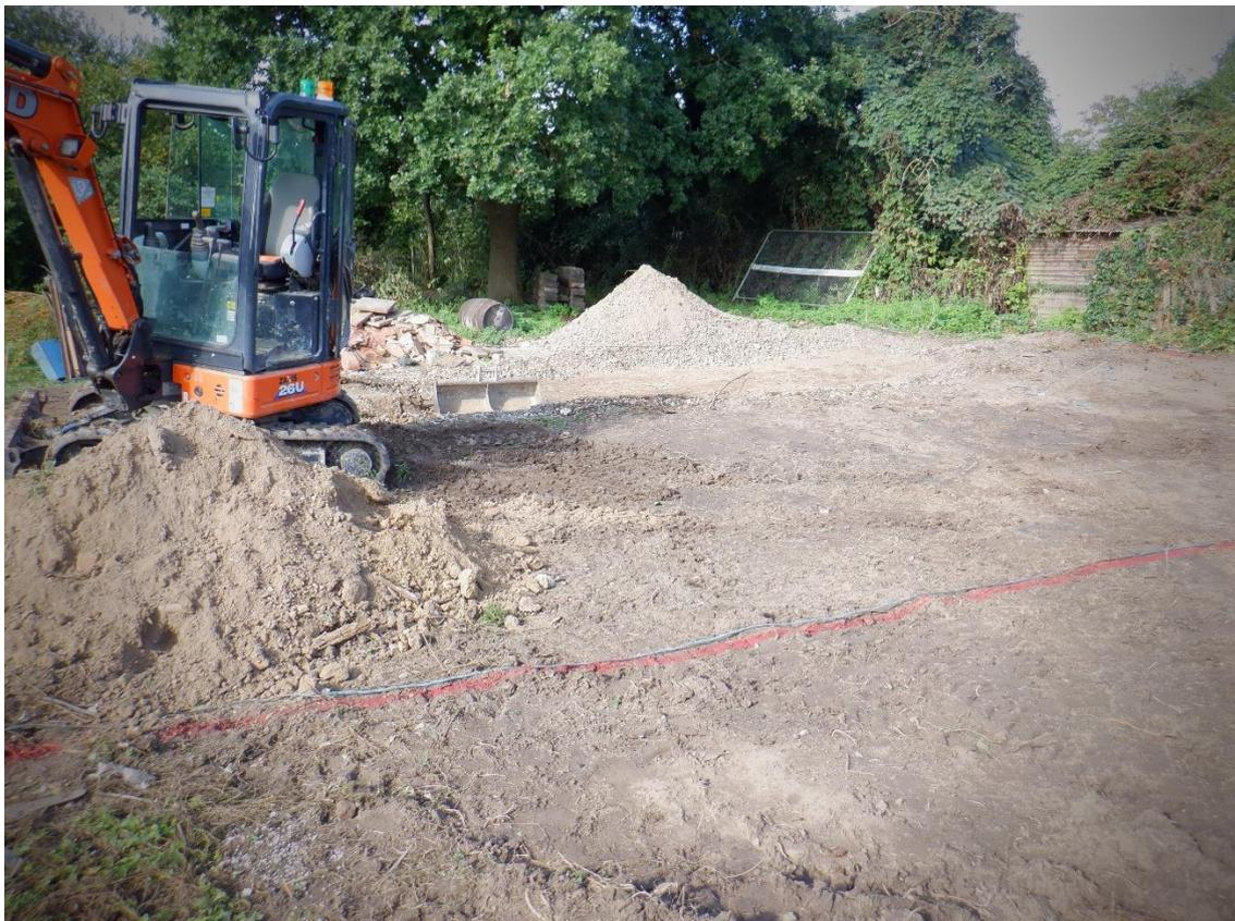
Plate 1. Setting out and starting ground reduction (looking SW)
