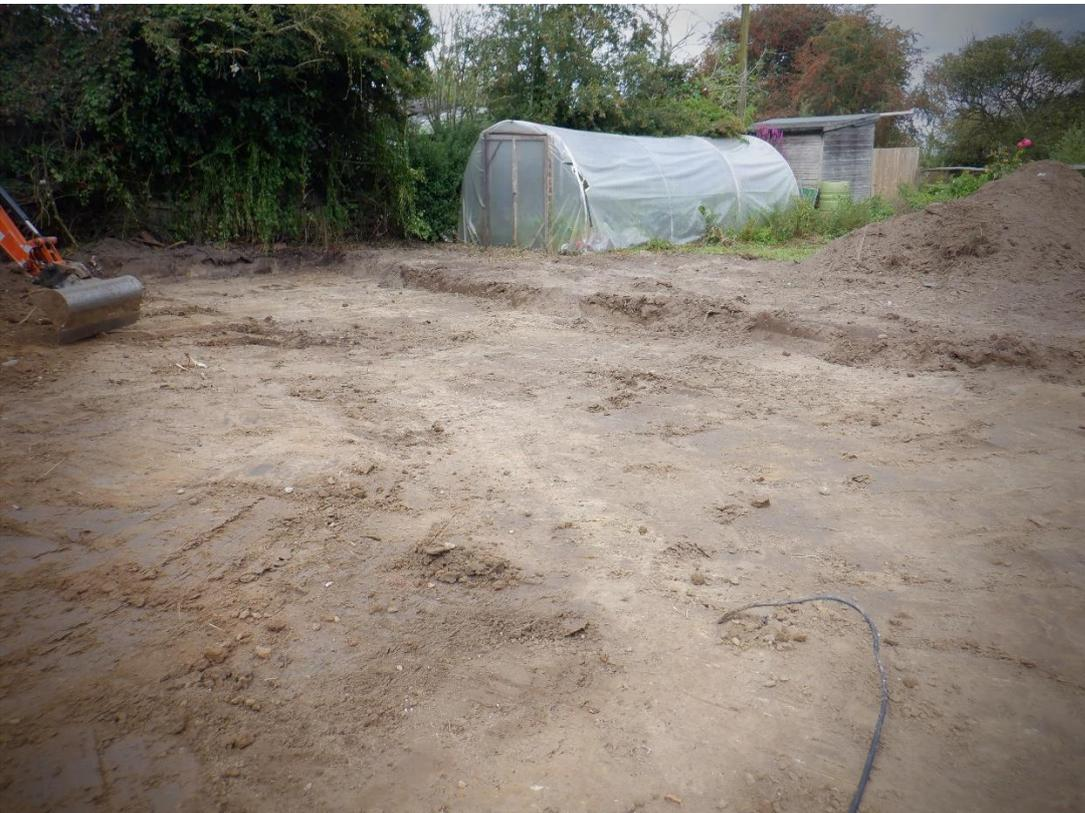
Plate 5. Ground reduction completed (looking North)
