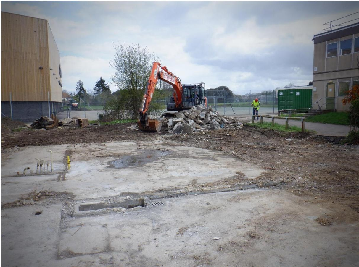
Plate 1. Removing concrete foundations and surfaces (looking North)
