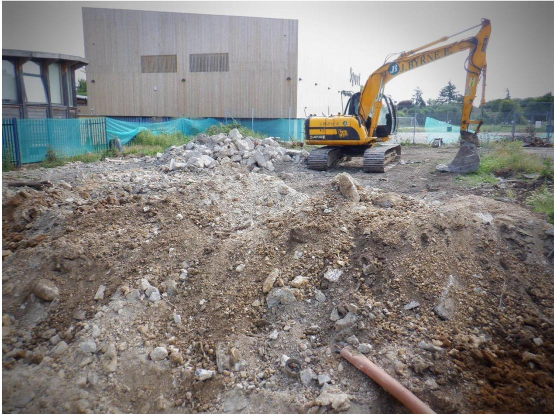
Plate 3. Removing foundation footing (looking NNW)
