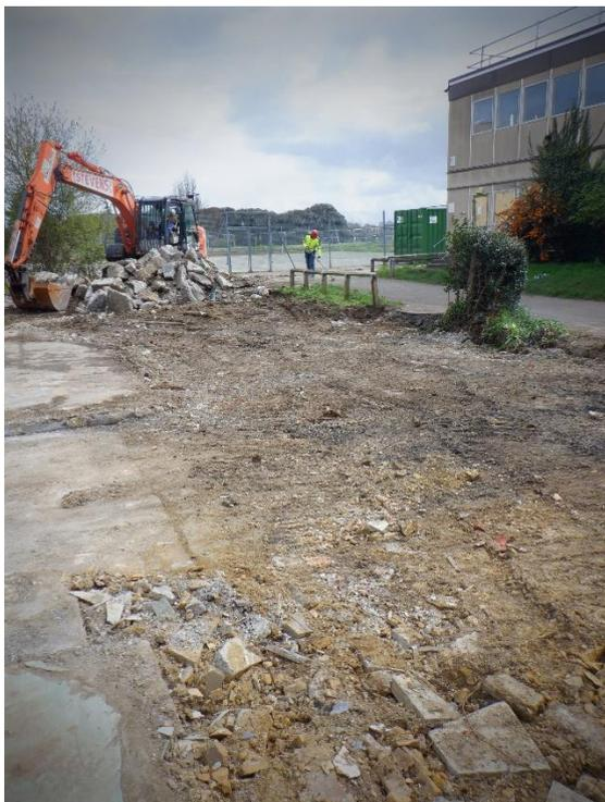
Plate 2. Removing concrete surfaces (looking North)
