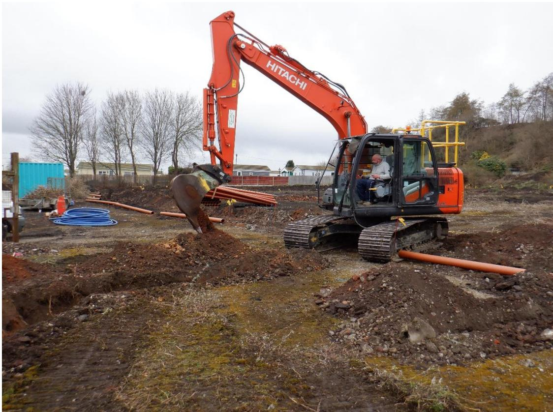
Plate 2. Service pipe run trenching (looking West)
