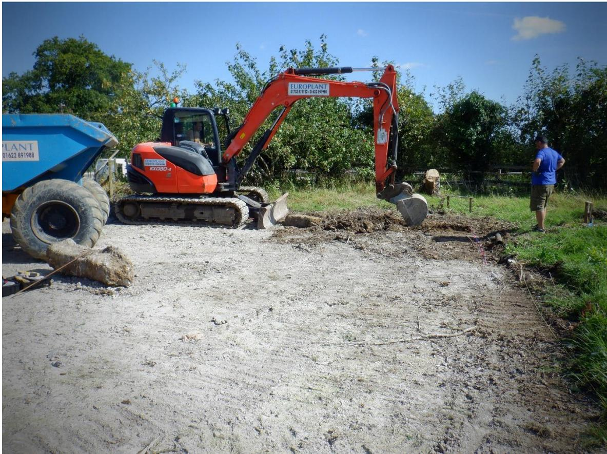
Plate 1. Removing grass and topsoil surfaces (looking SE)
