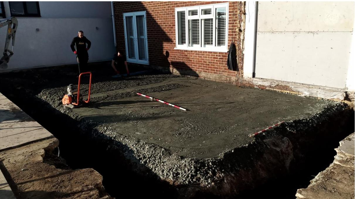
Plate 2. Foundation footings cut and stabilising tarmac surface(looking NW)
