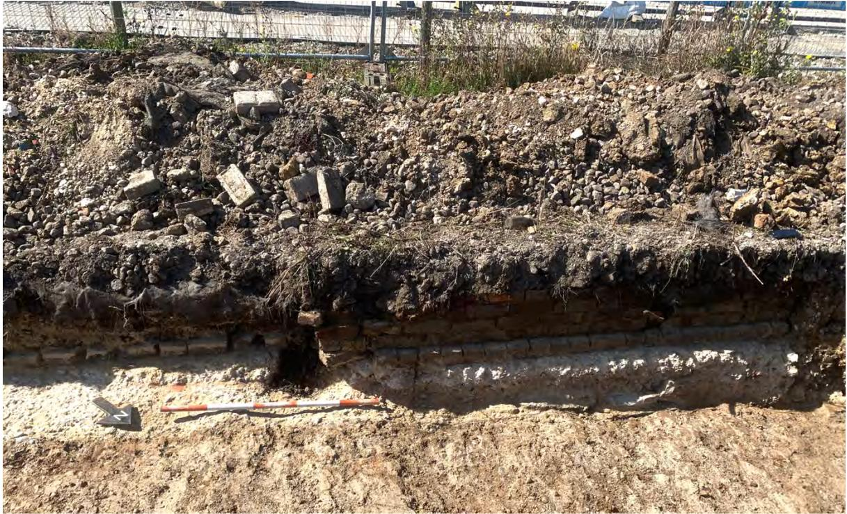
*Plate 8 Section showing brickwork (811) and (812) on concrete foundation (810)*
