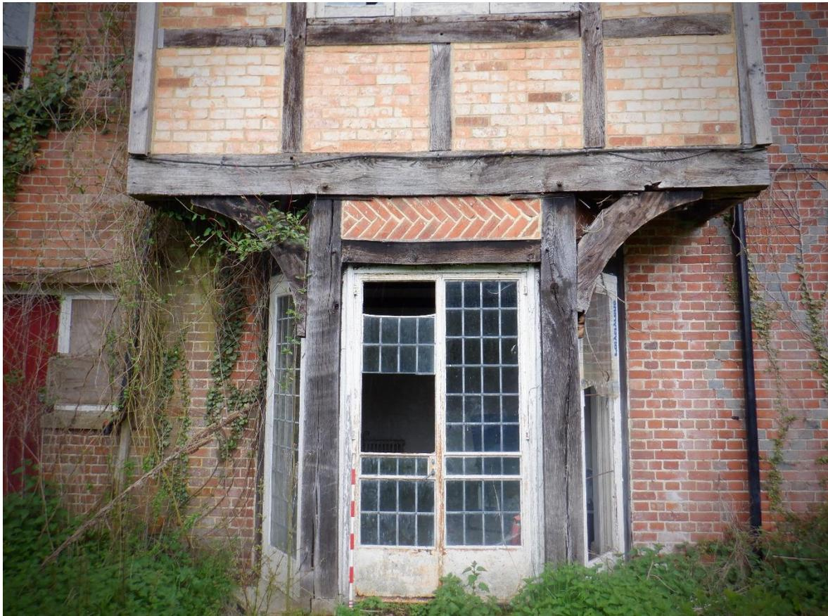
Plate 12. Detail of timber framed extension on NE façade (1m scale)
