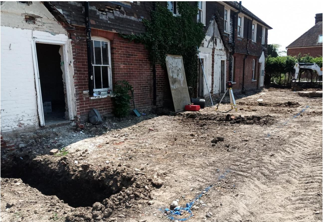
Plate 2: Foundations excavated in the eastern part of the site.
