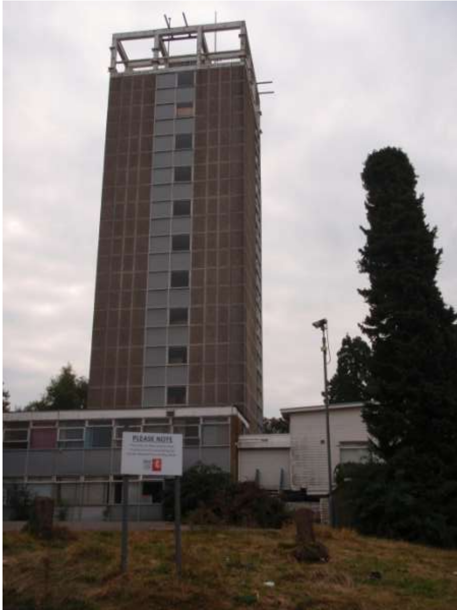
Plate 1. The exterior of the Tower Block. Column and Beam construction with factory produced external panels. All 11 floors were used as a book depository with 'Music' on Floor 2 to 'Classic Fiction' on Floor 11.
