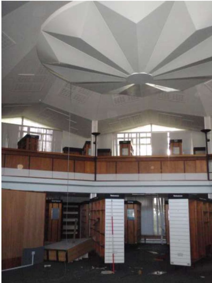
Plate 14. View of ground floor and upper floor of the library. The library is a polygon built design, again a modular build with the ground floor bookshelves radiating out and capped by an upper gallery with access by two timber open tread staircases
